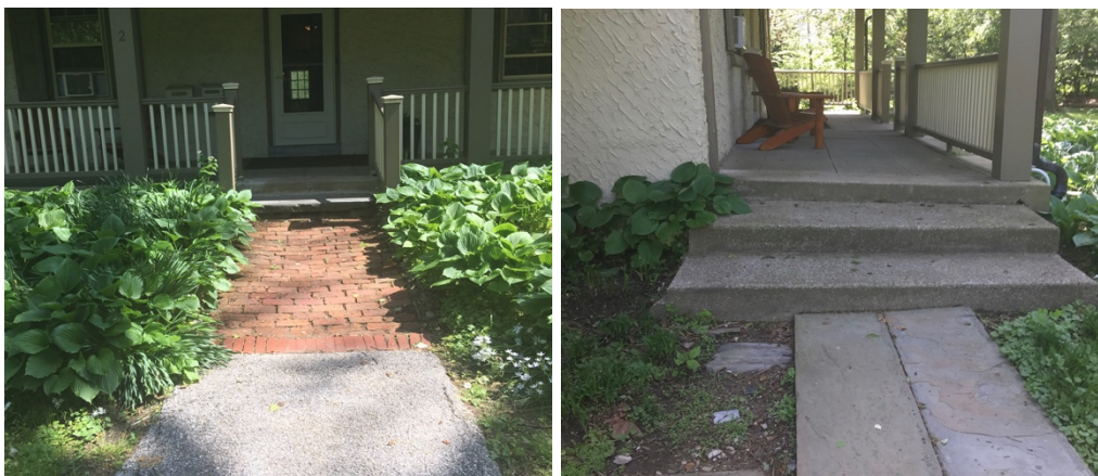
The inaccessible main entrance to Woodside Cottage, and a possible location for a ramp.
