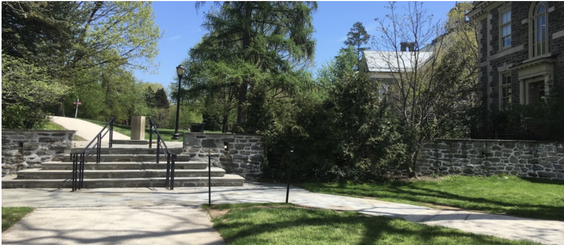
The inaccessible staircase that leads to Leeds and the playground.
