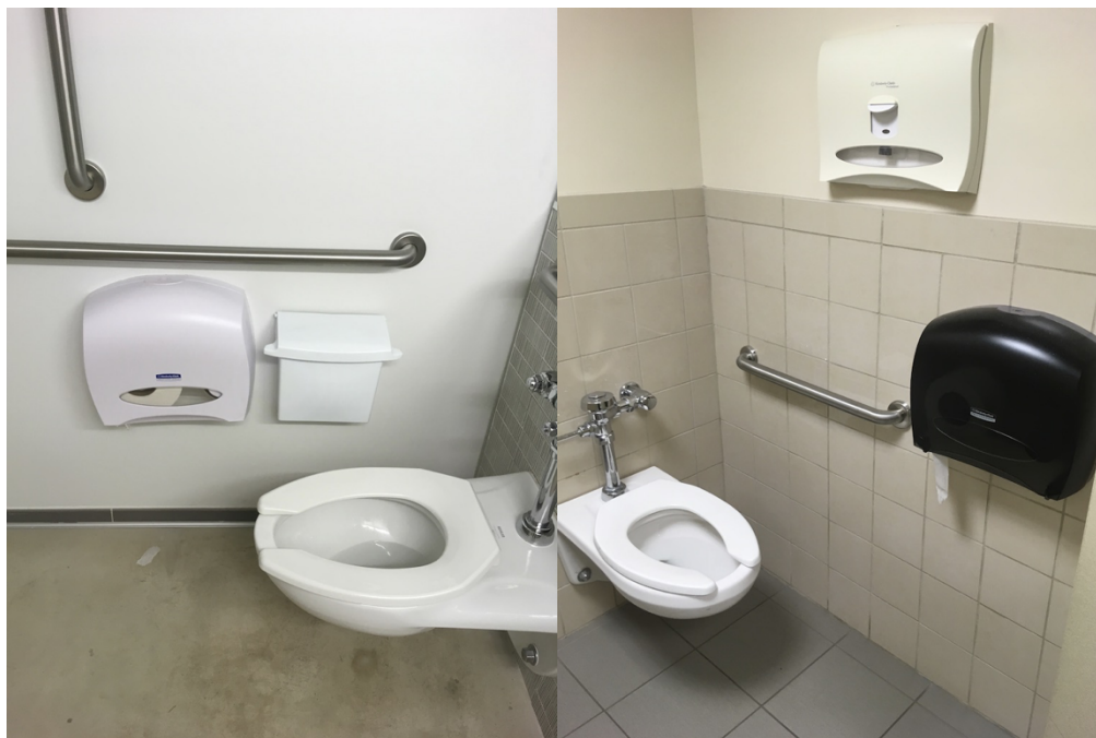
The accessible bathroom in the VCAM where the toilet paper is difficult to reach. (right)
